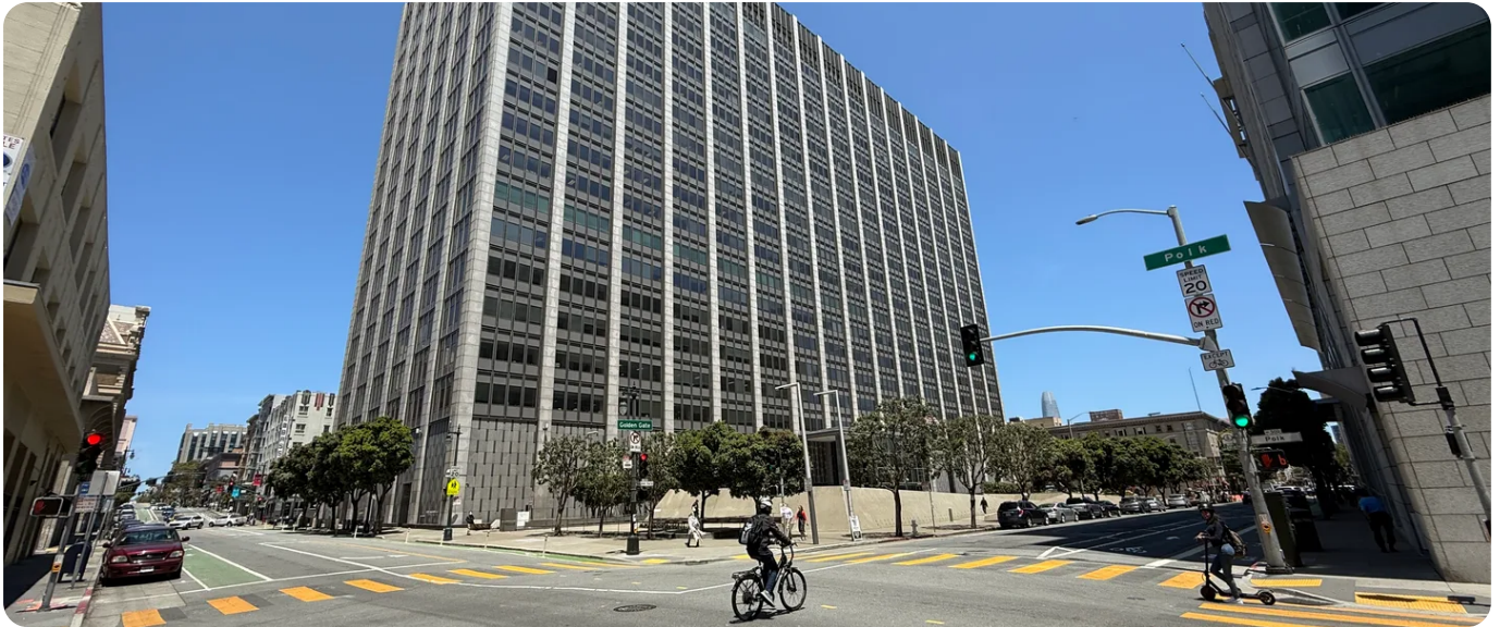
Phillip Burton Federal Building & United States Courthouse — Marincyclist, CC BY-SA 4.0, via Wikimedia Commons — recadrage et optimisation Law Right. Wikimedia Commons
